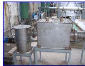
Air Cooling unit with out-let filter
