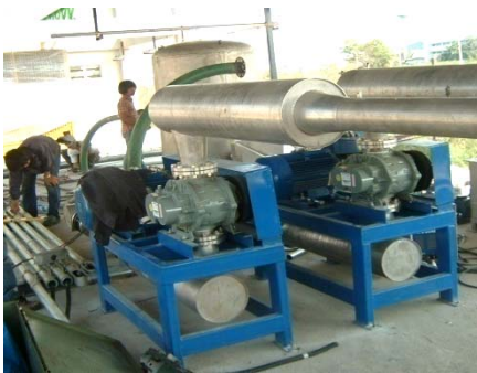
Installation on site
