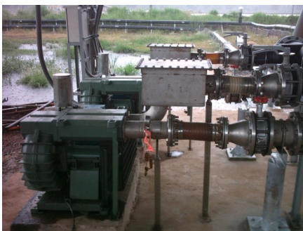
Central air supply system for gas burner
