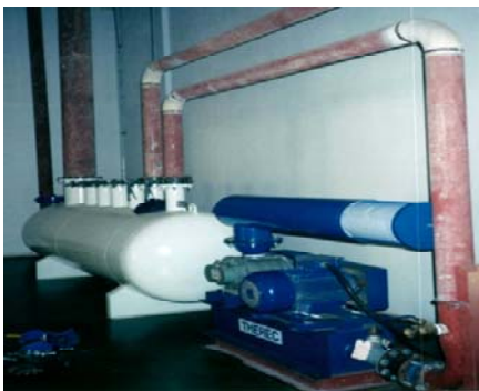
Central air supply system for gas burner
