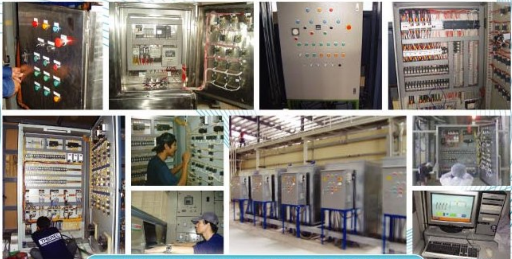
Capability in doing design, assemble and commissioning
